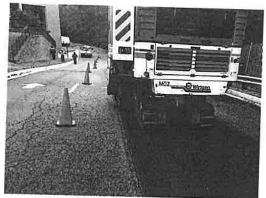
Full milling, curb to curb
