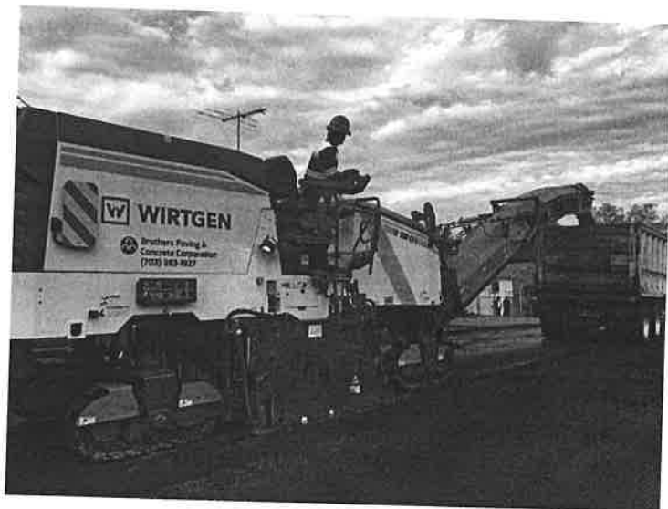
Milling entire parking lot
