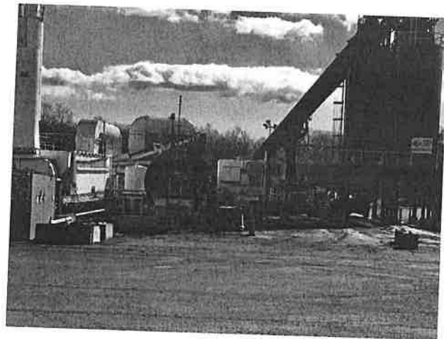
New asphalt materials made
