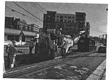
Milling in center of a four lane highway
